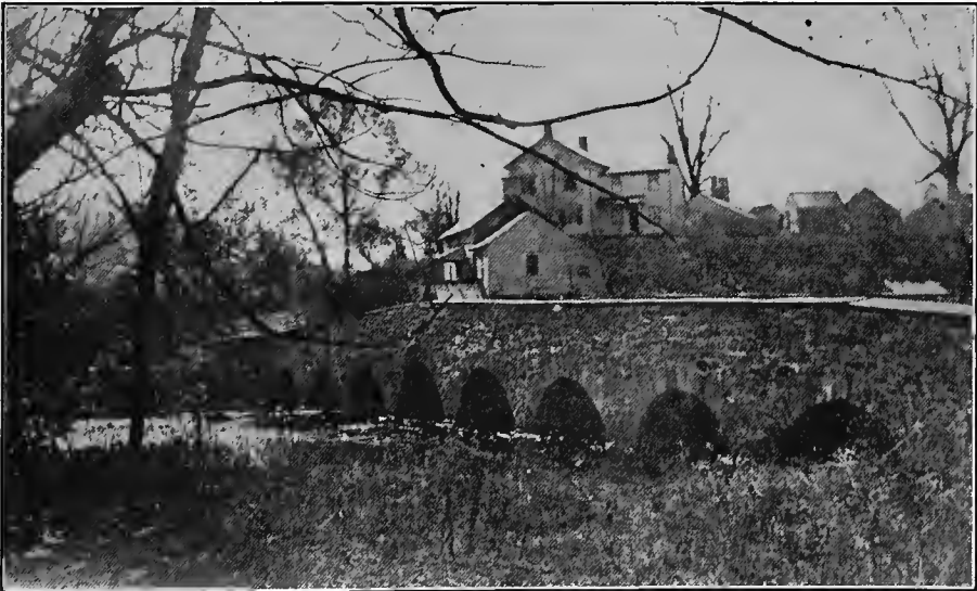
Stone Bridge built in 1836 at Bridgeville.
