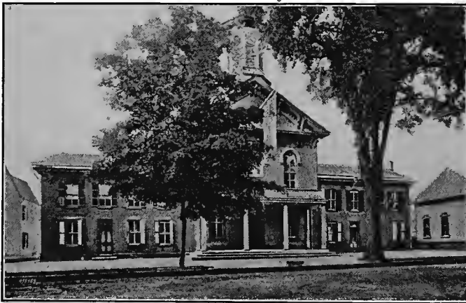
Warren County Court House, Belvidere.
