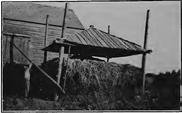
Raising a Barrack Roof.
