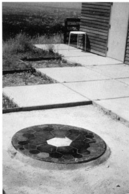
Fig. 3. Circle Limit 7 , the hyperbolic tiling of heptagons installed and curing at MSRI. The earthquake-stabilization hole in the middle is not yet drilled into the concrete pad and footings
