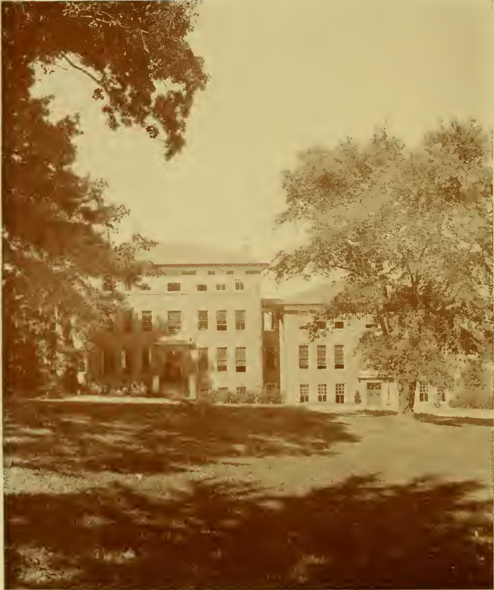
A PORTION OF THE ENGINEERING GROUP
