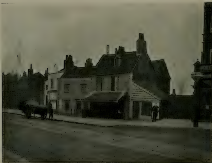
PLATE 42.—OLD HOUSES NEAR THE "WHITE HART" (NOW NOS. 168 TO 178).
