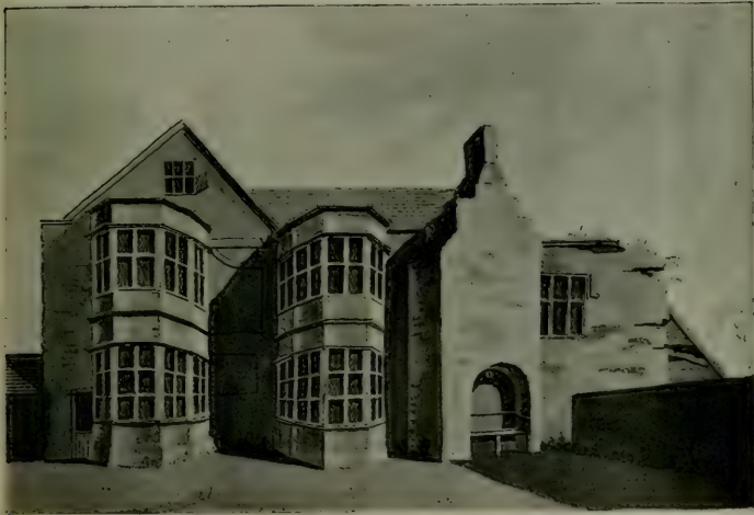
PLATE 66.—PLACE HOUSE, CATFORD, ABOUT 1810.
