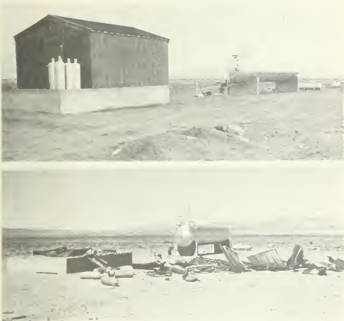
Figure 5.120. Upper photo: LP-gas bulk storage and filling plant before a nuclear explosion. Lower photo: The plant after the explosion (5 psi peak overpressure).
