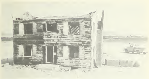
Figure 5.64. Strengthened wood-frame house after a nuclear explosion (4 psi peak overpressure).
