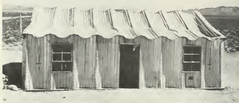
Figure 5.44. Self-framing corrugated steel panel building after a nuclear explosion (3.1 psi peak overpressure).
