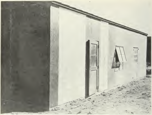
Figure 5.40a. Exterior of self-framing steel panel building before a nuclear explosion, Nevada Test Site.
