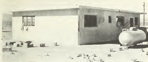
Figure 5.73. Reinforced precast concrete house after a nuclear explosion (5 psi peak overpressure). The LP-gas tank, sheltered by the house, is essentially undamaged.
