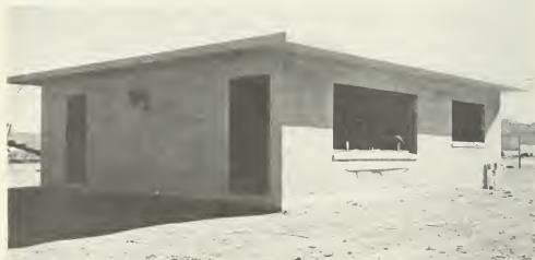
Figure 5.77. Reinforced masonry-block house after a nuclear explosion (5 psi peak overpressure).
