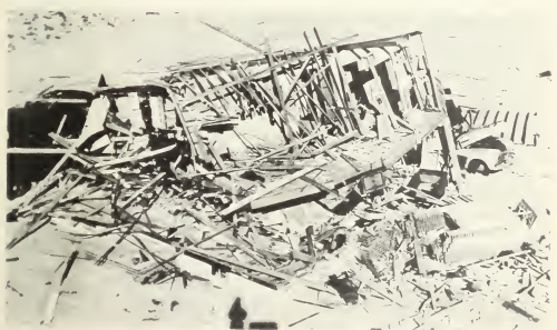
Figure 5.57. Wood-frame house after a nuclear explosion (5 psi peak overpressure).
