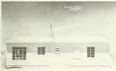
Figure 5.69. Rambler-type house before a nuclear explosion, Nevada Test Site. (Note blast door over bathroom window at right.)
