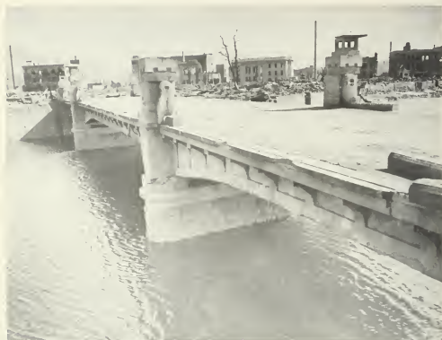
Figure 5.127a. Bridge with deck of reinforced concrete on steel-plate girders; outer girder had concrete facing (270 feet from ground zero at Hiroshima). The railing was blown down but the deck received little damage so that traffic continued.
