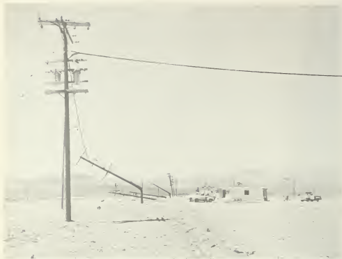
Figure 5.104. Collapse of utility poles on line (5 psi peak overpressure, 0.6 psi dynamic pressure from 30-kiloton explosion), Nevada Test Site.
