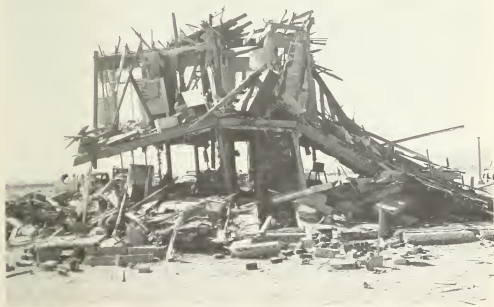
Figure 5.67. Unreinforced brick house after a nuclear explosion (5 psi peak overpressure).
