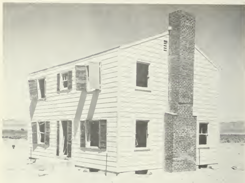
Figure 5.65. Strengthened wood-frame house after a nuclear explosion (2.6 psi peak overpressure).
