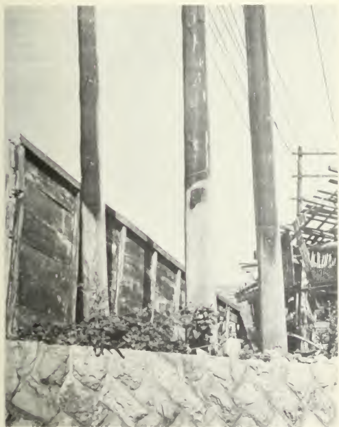
Figure 7.44b. Flash burns on wooden poles (1.17 miles from ground zero at Nagasaki, 5 to 6 cal/cm 2 ). The uncharred portions were protected from thermal radiation by a fence.
