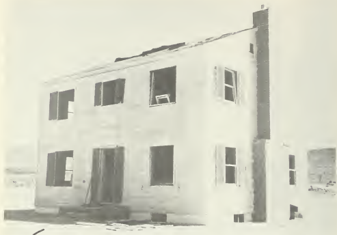
Figure 5.59. Wood-frame house after a nuclear explosion (1.7 psi peak overpressure).
