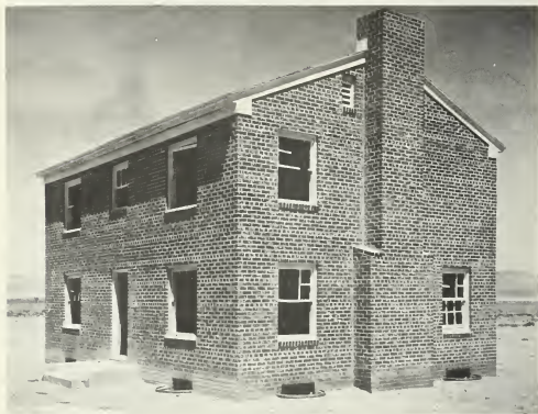
Figure 5.68. Unreinforced brick house after a nuclear explosion (1.7 psi peak overpressure).
