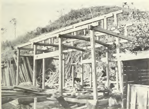
Figure 5.52. Upper photo; Wood-frame building; 1.0 mile from ground zero at Hiroshima. Lower photo: Frame of residence under construction, showing small tenons.
