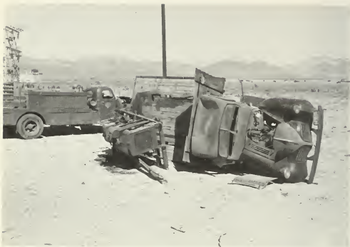
Figure 5.89. Truck broadside to the blast wave (5 psi peak overpressure) overturned; electric utility truck in background head-on to blast was damaged but remained standing.
