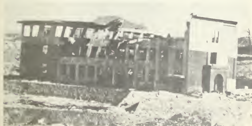
Figure 5.22b. Effects of horizontal loading on wall facing explosion (0.4 mile from ground zero at Nagasaki).
