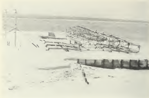
Figure 5.51a. Structure similar to Figure 5.48a after exposure to 6.1 psi peak overpressure and 0.6 psi dynamic pressure; positive phase duration several seconds.
